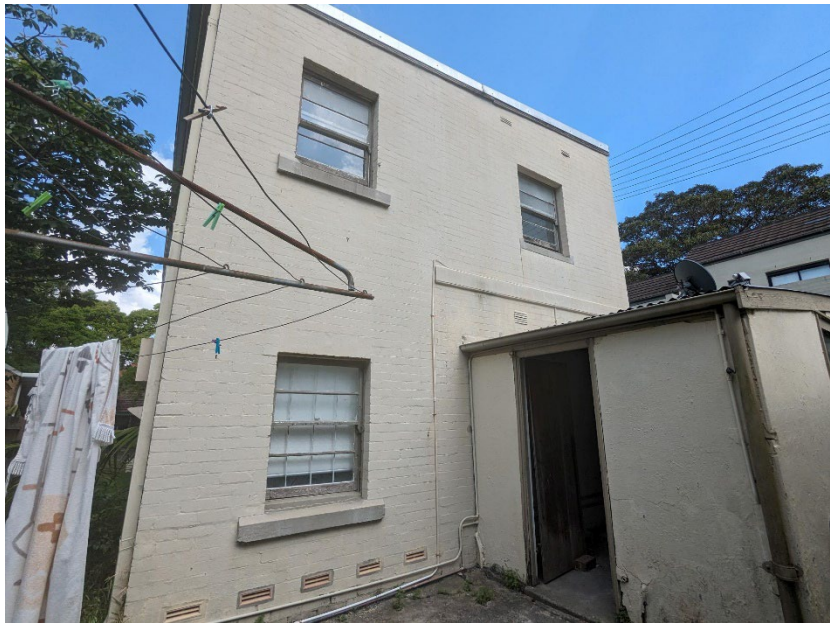
rear elevation and storeroom
